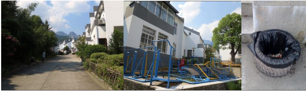
Figure 5 Road and greening
